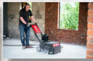
Grinding Concrete
