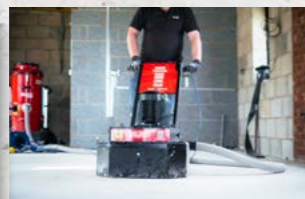
Removing High Spots
