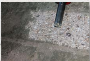
Roughening Concrete
