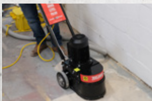
Grinding Concrete
