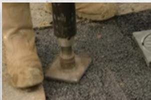
Asphalt Compaction
