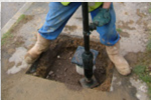
Reinstatement Compaction
