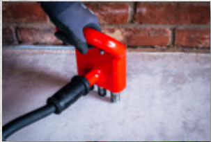
Reducing Levels on Concrete
