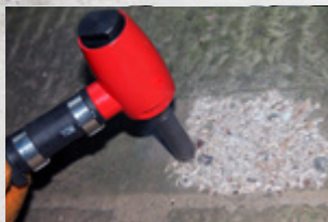
Reducing Levels on Concrete
