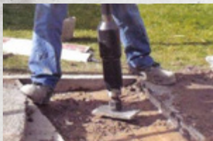
Back Fill Compaction
