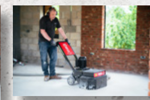
Grinding Concrete
