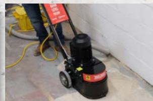
Grinding Concrete
